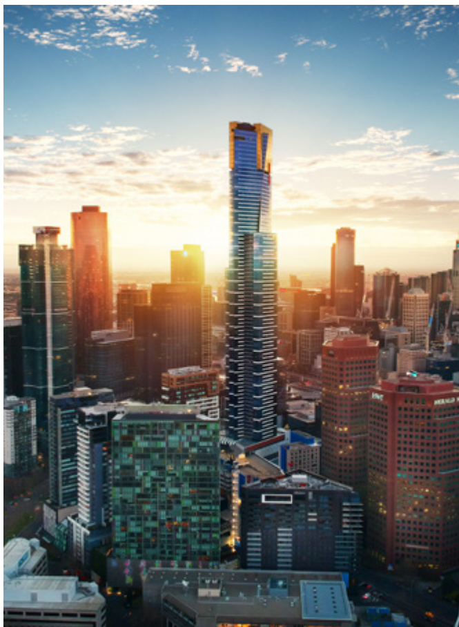
EUREKA TOWER, MELBOURNE, VIC
